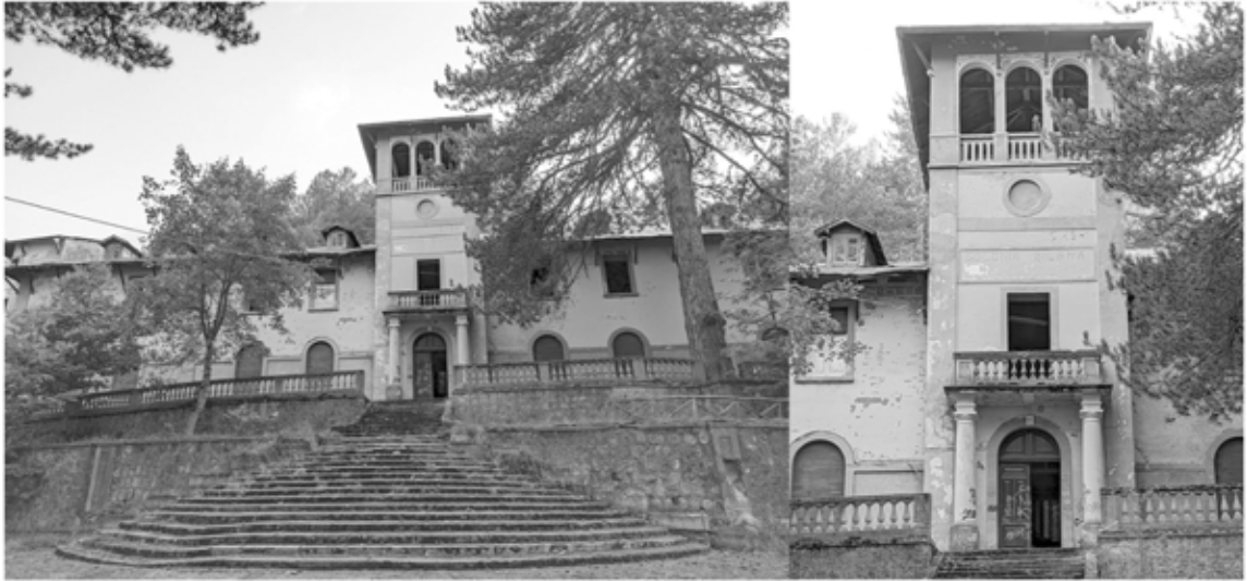
Figure 3: The main building, façade and a detail (photo by Alfonso Morelli - Team Mistery Hunters)
