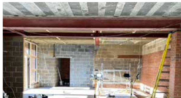
Building work commences
