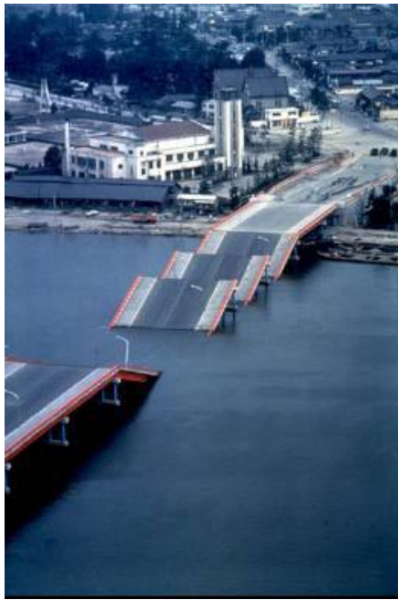
Figure 19(a): Collapse of Showa bridge, 1964 Niigata earthquake, Japan. Photo courtesy: NISEE website.
