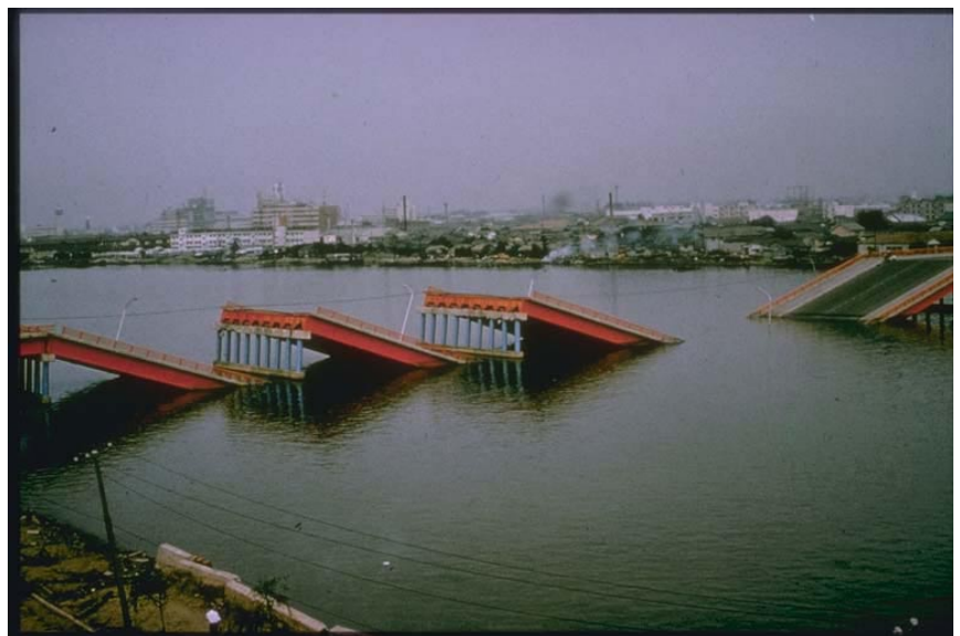
Figure 19 (d): Another view of the collapsed bridge. The figure shows the foundation system. Photo courtesy: EERC (University of California) website.
