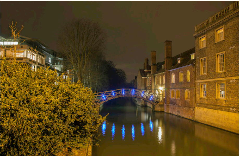
A Light Installation on the Mathematical Bridge. Photo: Dr Brian Callingham.
