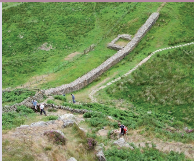
View of Hadrian's Wall, close to the problematical turret 'Peel Gap' in Wall Mile 39.
