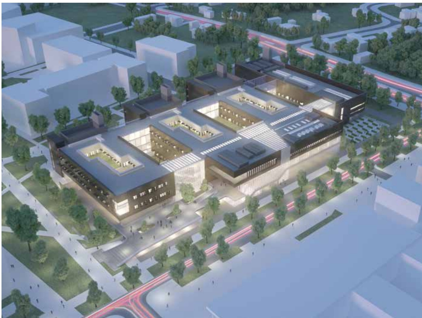
Fig.3. The research and teaching wings are connected together by parallel north-south corridors on all levels. As well as giving very good connectivity across the site these corridors also enclose the internal courtyards, which will provide a pleasant outlook for the offices surrounding them. The research wings also have smaller courtyards set into the upper floor, which should create an excellent environment in the areas with high densities of offices.
