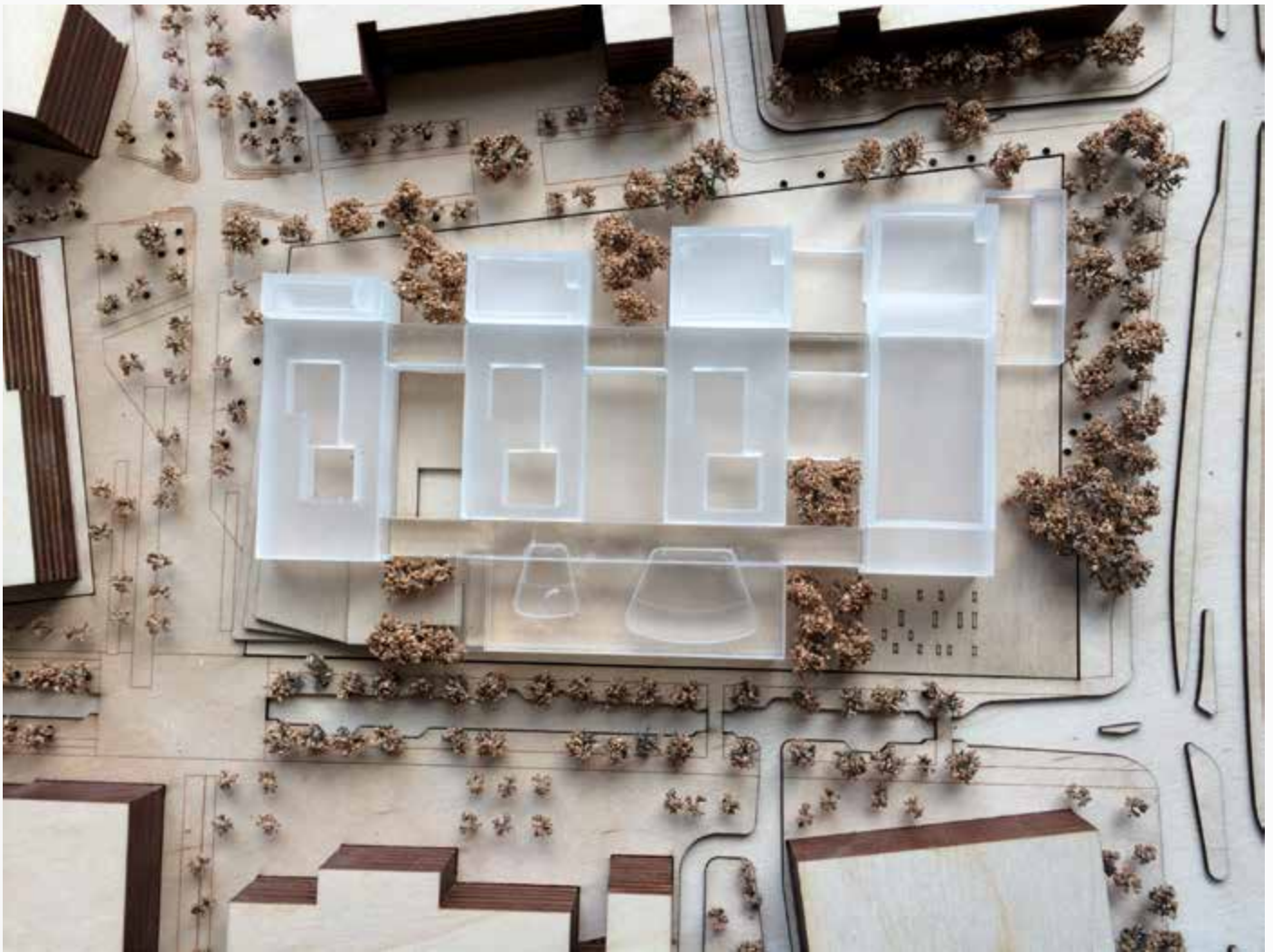
Fig. 2. A model of the building layout shows how the new building fills the Paddock site. Madingley Road is at the right, and J.J. Thomson Avenue at the bottom. The main entrance lies on J.J Thomson Avenue, and gives direct access to an open area housing two lecture theatres as well as an exhibition area. To the south (left) there will be a pleasant open area separating the Cavendish from another new building which will house many communal facilities including a full-scale canteen.
