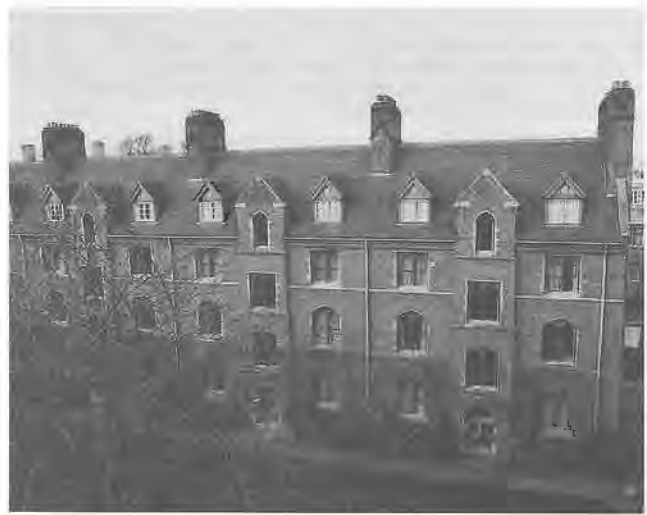
Friars Building from the Chapel Roof.
