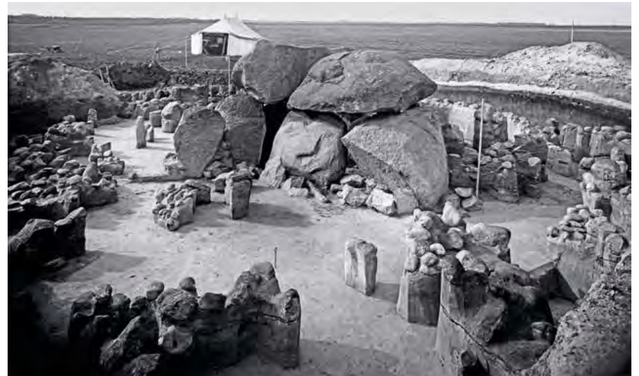
The excavation of tomb D40 in 1921. Over the years, Van Giffen developed his own standard excavation procedure in which the documentation of sections and surfaces was optimized
